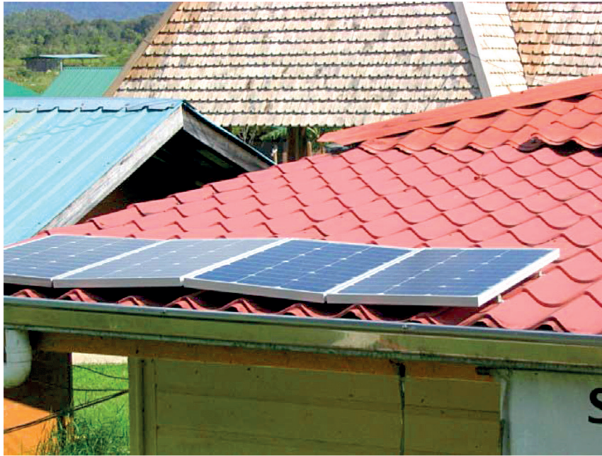
Figure 2-2-4: Solar panel installation on barrio telecentre's rooftop
