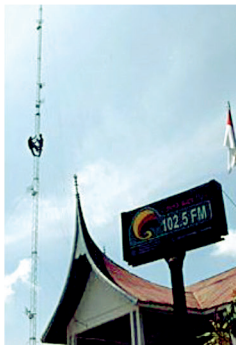
Antenna Unit Installation
