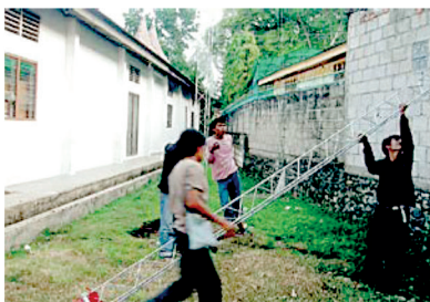
Preparation of Tower Installation
